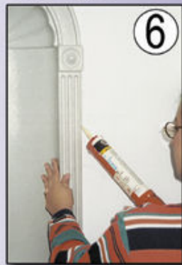
6 Caulk around edges (use paintable adhesive caulk)
