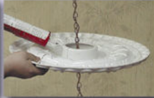
Caulk in points inside and outside edge (use adhesive paintable latex caulk).
