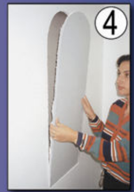
4 Cut and remove drywall
