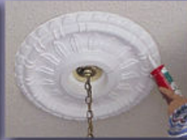
Caulk around crack, sand, prime and paint.
