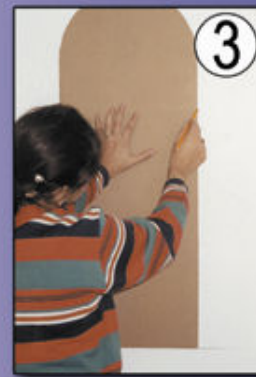
3 Trace template between studs
